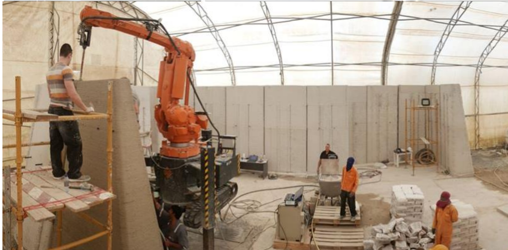
Tisk metodou FDM robotickým ramenem KUKA (IAAC, Institute for advanced Architecture Catalonia [online])
